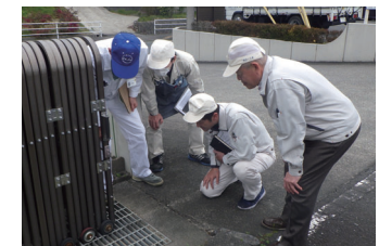
Checking the final drainage ditch witnessed by the business partner
