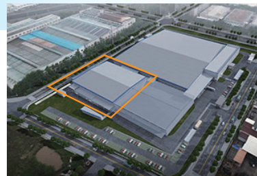
Foshan: Image of completed new building
